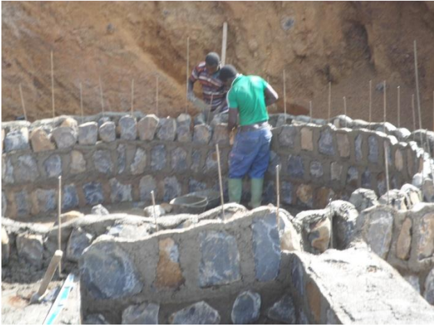
Storage Tank construction in Progress
