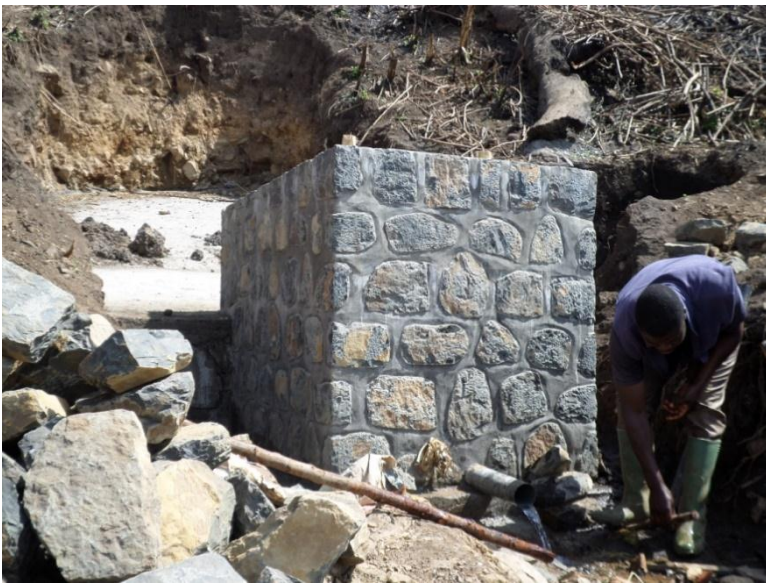
Catchment Near Completion
