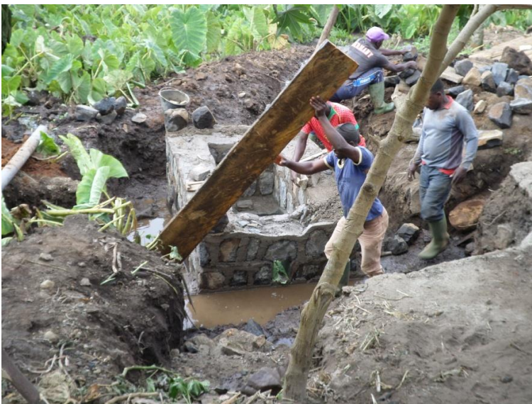
Spring catchment construction in progress
