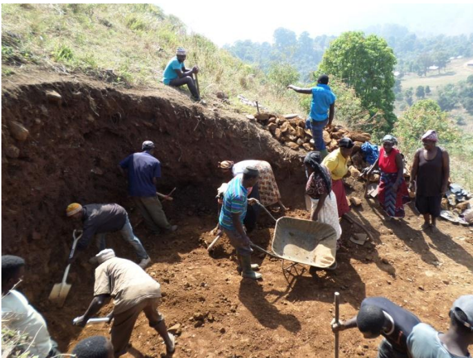
Community Works at Storage tank Site.
